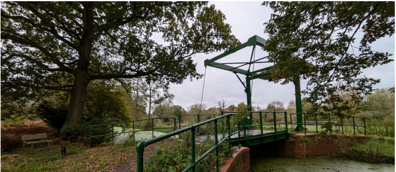
Birtley Lift Bridge no.1
